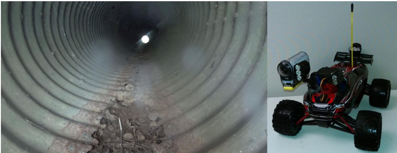
A. Image captured by HIVE on a 24" culvert under TH26 near Brownsville B. HIVE Vehicle
